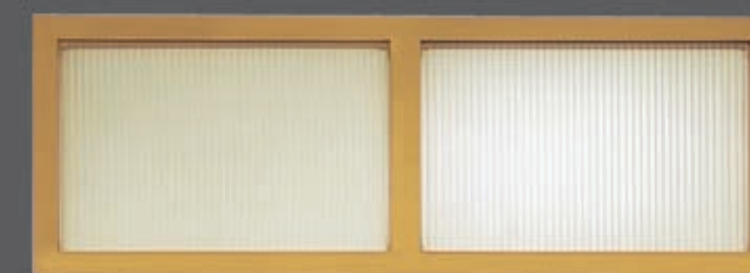
Sopraluce in policarbonato Polycarbonate fanlight
